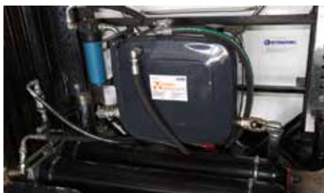
MISER pilot installation showing hydraulic storage.
